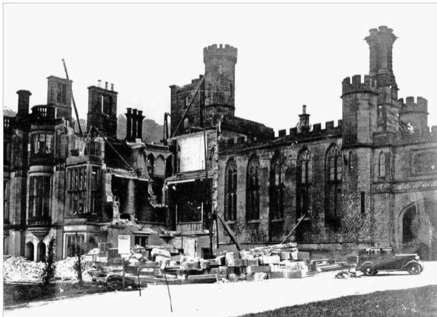
This facsimile print shows the Gothic pile in a state of deconstruction, probably in 1934. The demolished stonework lay in saleable heaps, and more was to be knocked down before the demolition was complete. No doubt the immediate availability of building materials made the partial reconstruction easier for the YHA and the National Trust (YHA Archive)
