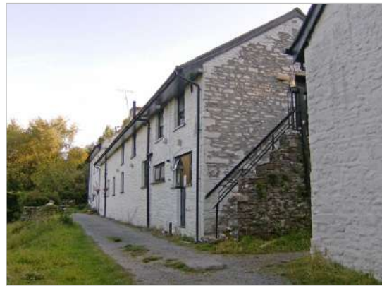
The crooked straight: the 1992 work at Llwyn-y-Celyn remedied severe wall bulges and a defective roof. 1&2: the original structures, as photographed in the 1970s – looking south and north respectively (YHA Archive); 3&4: by contrast, the same buildings about 20 years later. Note the swapped positions of the entrance door and adjacent window in the farmhouse, the infilling of arch-topped barn entrances and the blanking off of another door. The later staff and guest accommodation known as the Annexe is nearest in image 4 (author's images, September 2015)
