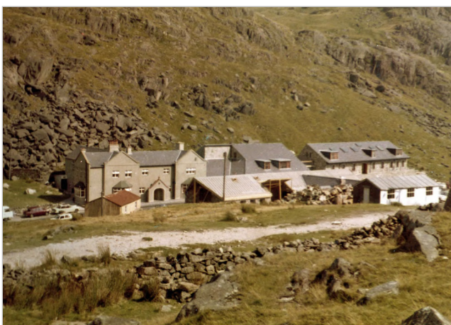
The new hostel and restaurant take shape – 1: the restaurant under breeze block, glass and timber construction; 2: the new long barn (the date is probably 1971, as the Car Park charges are portrayed both in shillings and new pence); 3&4: old huts still jostle for space alongside the newly emerged restaurant (photographs by Max Kirby, YHA Archive)
